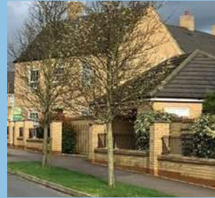
Low walls with piers and rails
