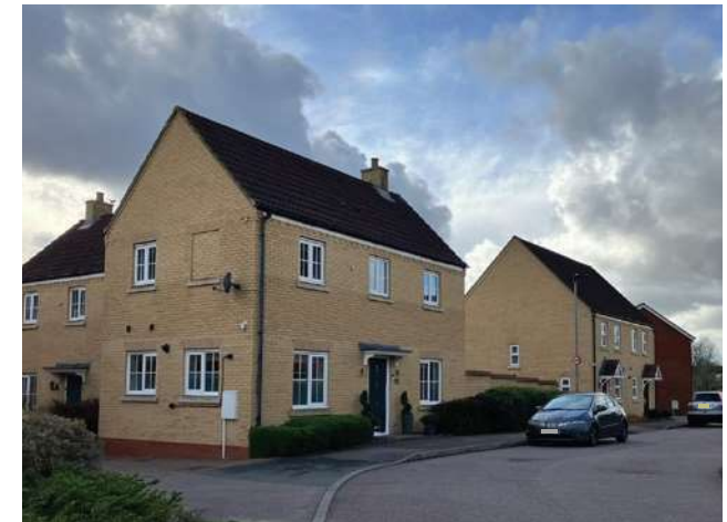
Figure 31: Denser suburban housing in the Aspires development.
