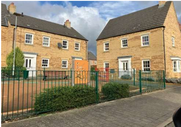
Figure 32: Small surfaced recreation and play area in front of homes on the corner of Primrose Fields.
