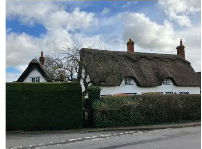
Figure 35: Thatched cottage with eye-brow dormers is an example of the rural settlement heritage.
