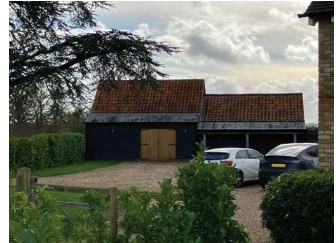
Figure 61: Example of side of plot parking with characterful carports and hedges that screen parking.
